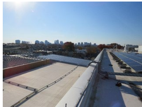
Harrison HS - Building Envelope
